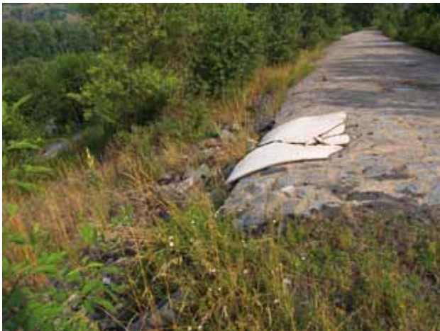
Fig. 7. Remains of the old, sealed embankment, and below the new, loose assemblage of rocks. Photo: MIKULÁŠ VELENSKÝ
